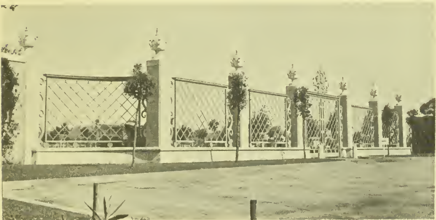
Main Entrance Gate.
